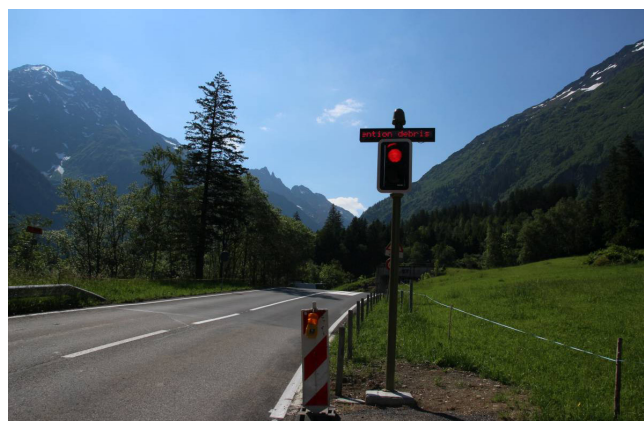
Figure 3: Several traffic light automatically close the road in case of an event. Further information on the closure reason is displayed for the waiting motorists.
