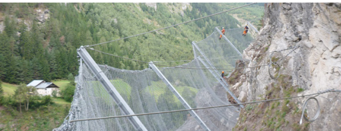
Title Page: Sensors above the construction site near Ovella.
