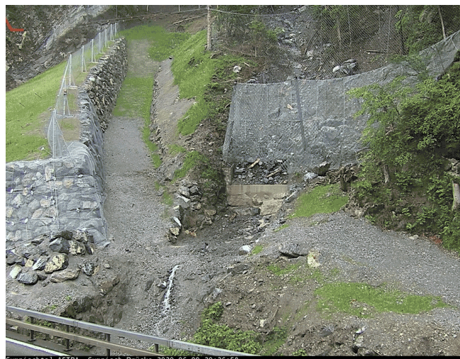
Figure 4: Rockfall dam with attenuator protection net.
