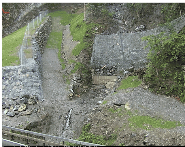
Figure 4 : Filets de protection.
