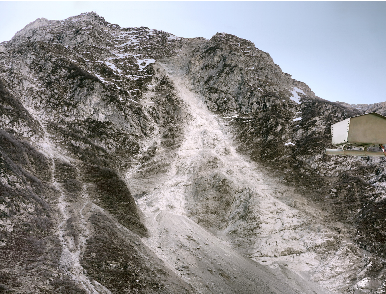
Deformation camera Ochsenstock, Switzerland
