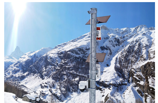
Avalanche radar with automatic road closure, Zermatt, Switzerland
